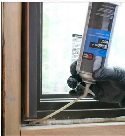
Available in a variety of sizes, HandiFoam low pressure polyurethane foam sealants are designed to seal and fill small gaps, cracks and voids and can be applied with a professional dispensing unit. HandiFoam sealants cure when ambient moisture/humidity in the air reacts with the foam sealant creating a rigid, closed cell barrier against drafts, noise, moisture and air infiltration.
