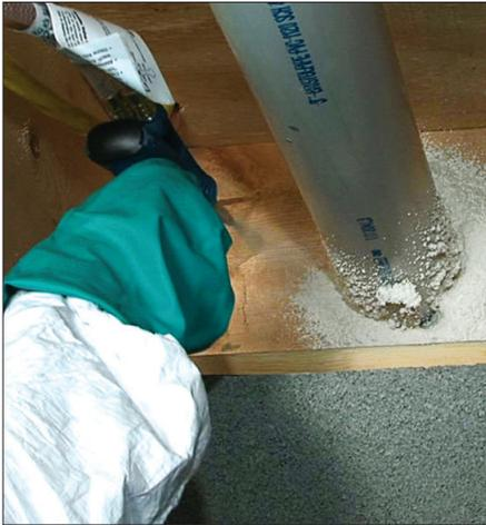
Available in a variety of sizes and formulations, HandiFoam® low pressure spray polyurethane foams are specifically designed to fill large voids and surfaces, creating a monolithic seal. HandiFoam spray polyurethane foams are often used to stop air infiltration and complete the building envelope. This helps improve indoor air quality, lower heating and cooling costs and drastically reduce energy consumption.
